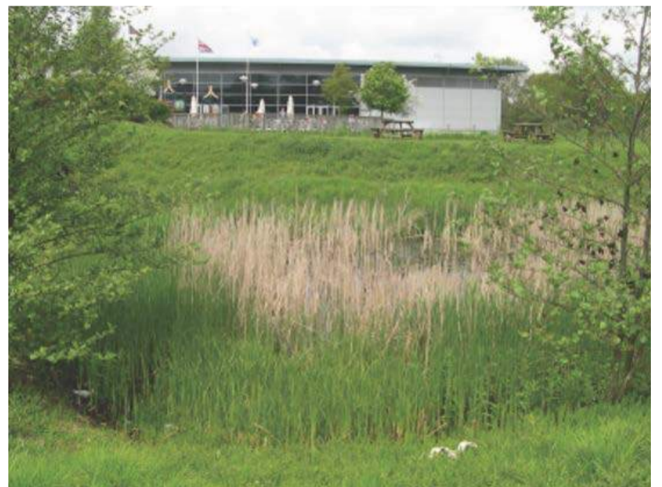
SuDS Pond/Wetland, Hopwood Service Area, M42
