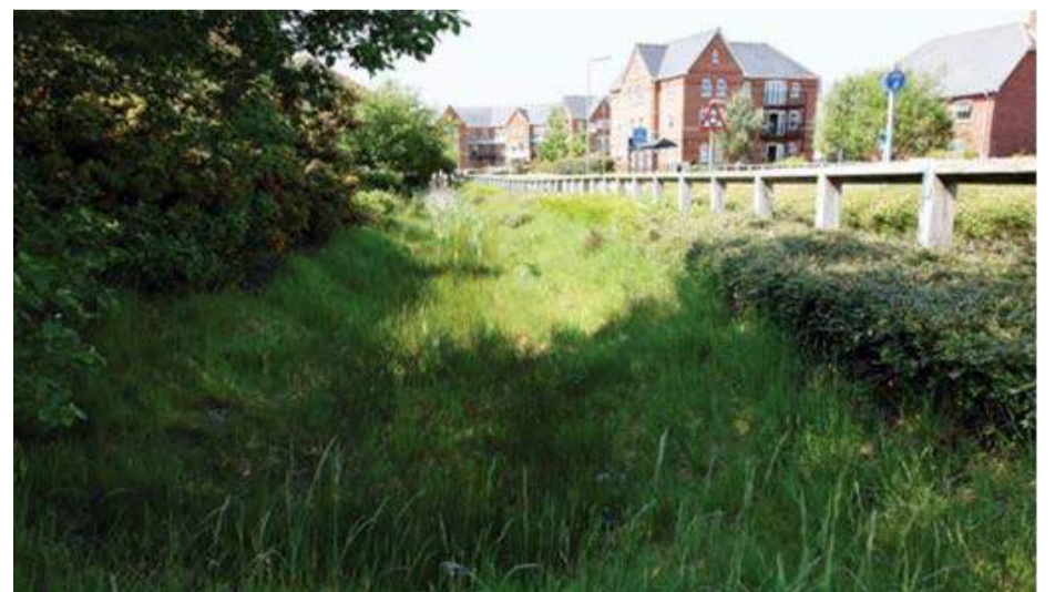
Roadside Swale, Elvetham Heath, East Hampshire
